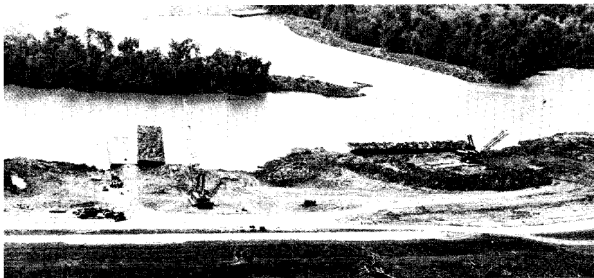
Building levees along the Atchafalaya River.
