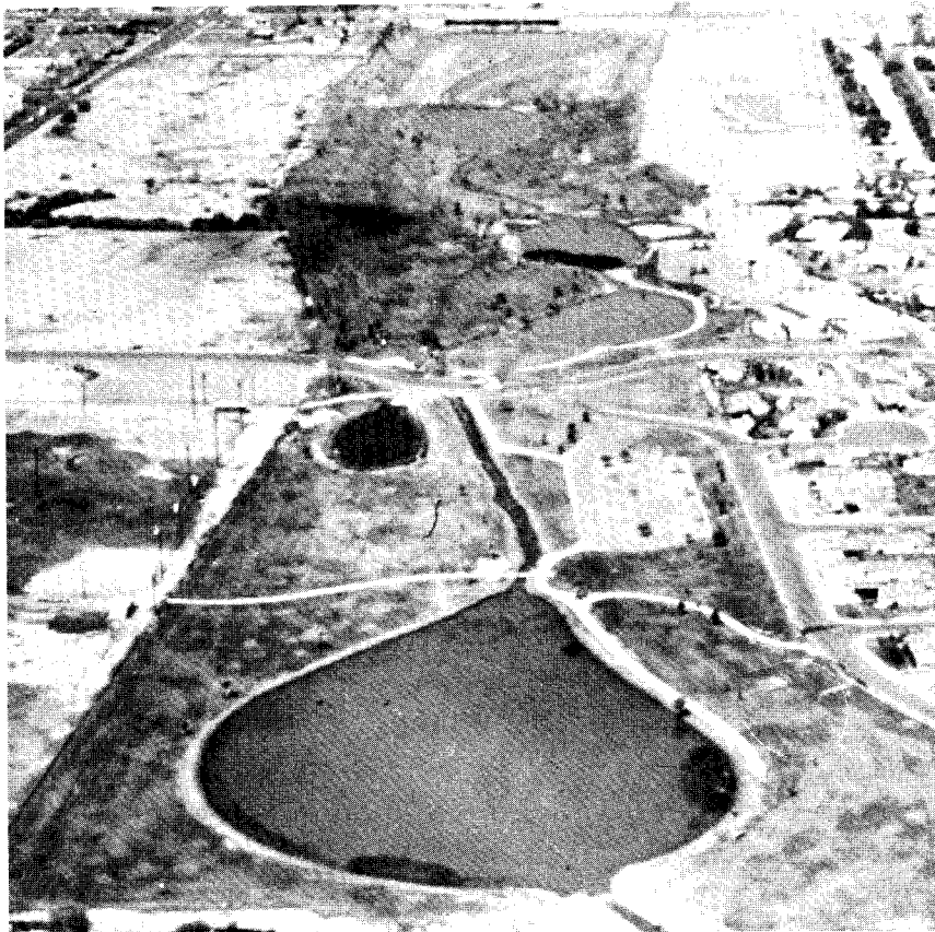
A nonstructural answer to flood control problems, Indian Bend Wash, Scottsdale, Arizona.
